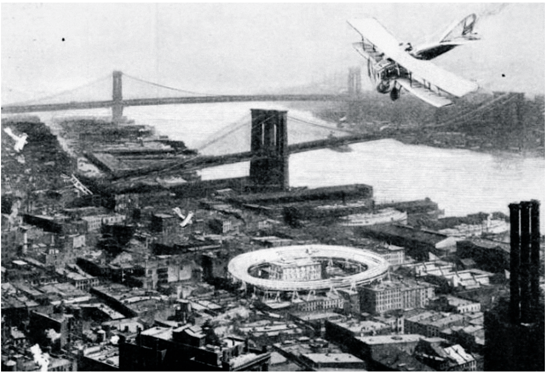
FIG. 2 A rooftop airstrip situated in the center of Manhattan, 1919. From Carl Diensbach, "Roosts for City Airplanes," The Popular Science Monthly (June 1919).
