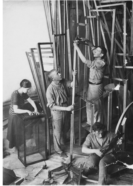
Model under construction. Petrograd. 1920.
