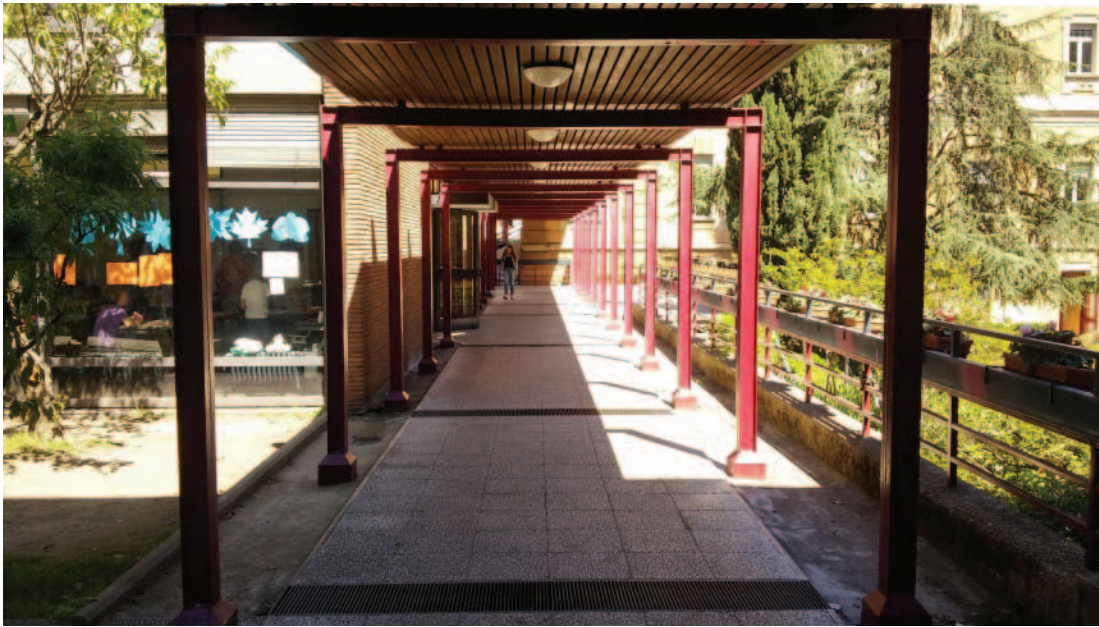
Fig. 1. The metallic arches of the Goethe-Institut portico. (© Claudio Panariello)
