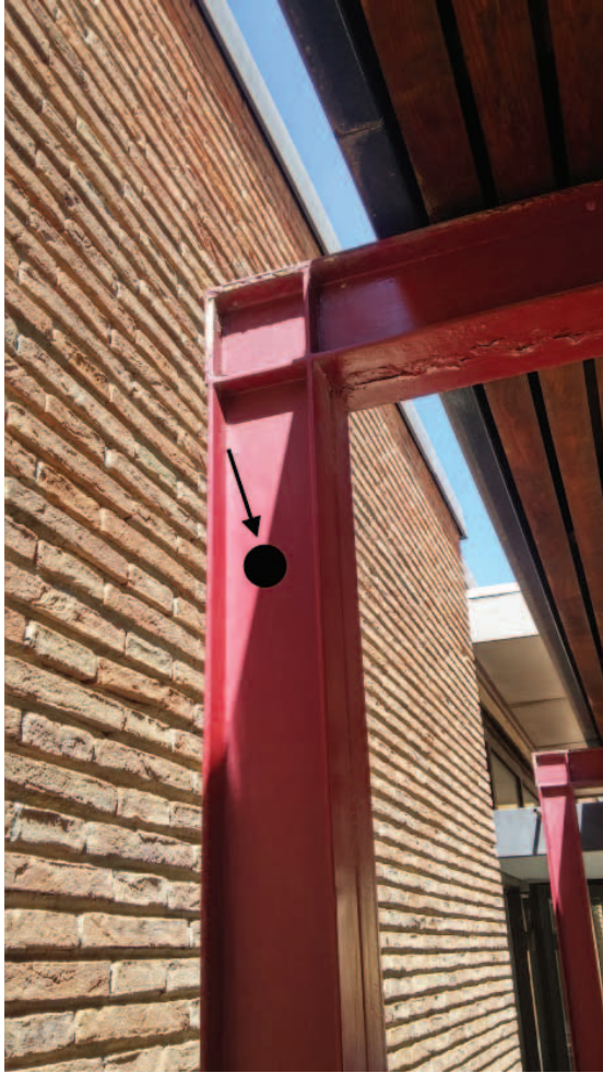
Fig. 3. Ideal resonating point on the vertical arch's pillar for the solenoid placement. (© Claudio Panariello)
