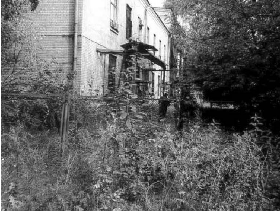
Figure 1. Moscow building with enough HEU for a bomb, 1994.
