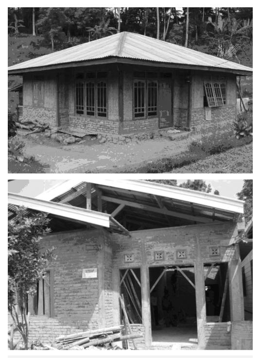
**Two common house types suitable for Haiti** *Top:* Timber frame with masonry skirt wall *Bottom:* Confined masonry, done well
